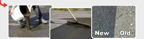
BORNIT®-Asphalt Pore Sealer - ready-to-use, solvent-free bitumen slurries with mineral additives, easy-to-process, quick-drying.
