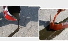
BORNIT®-Crack Flex - highly flexible polymer bitumen repair compound, solvent-free, weather- and UV-resistant, elastic after thorough drying, crack-bridging and highly adhesive at the substrate. Spreading of 2/5 highgrade chippings required.
