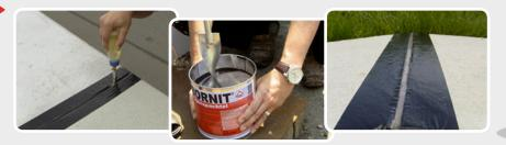
BORNIT®-Cold Sealing Compound / BORNIT®-Cold Joint Sealant -2-component polysulfide joint sealing materials, weather- and agingresistant; BORNIT®-Cold Sealing Compound (self-levelling) for horizontal joints or BORNIT®-Cold Joint Sealant (stable) for vertical and inclined joints, respectively. Priming with BORNIT®-Concrete or Asphalt Primer.
