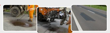
BORNIT®-Bitumenemulsion C60B5-REP - bitumen emulsion with fast breaking and setting behaviour in contact with high-grade chippings, solvent-free; following spraying, depending on the application, immediately spread suitable high-grade chippings.
